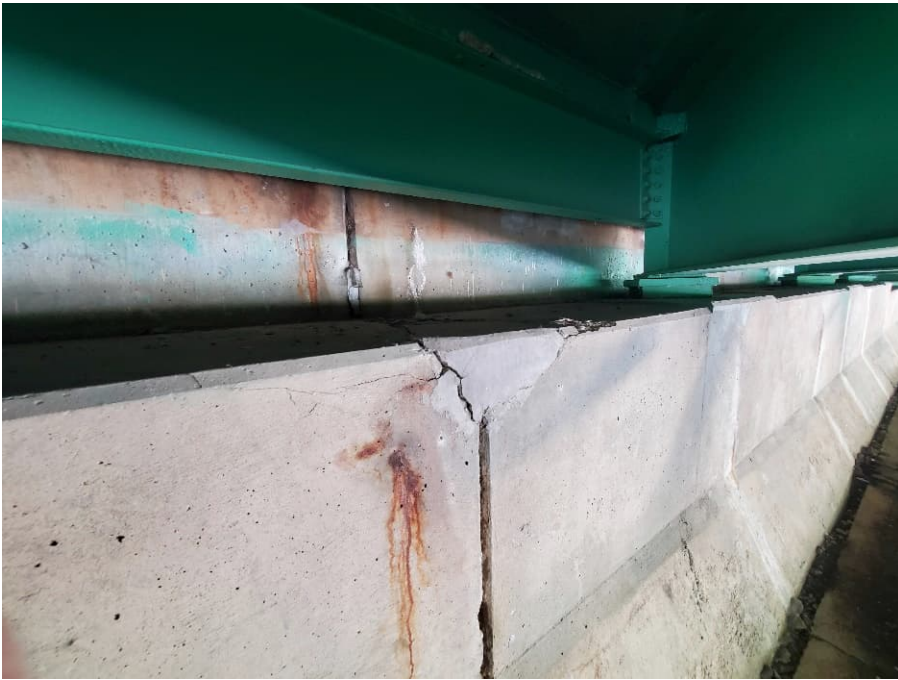
Abutment Damage
