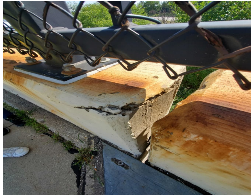
Parapet Damage
