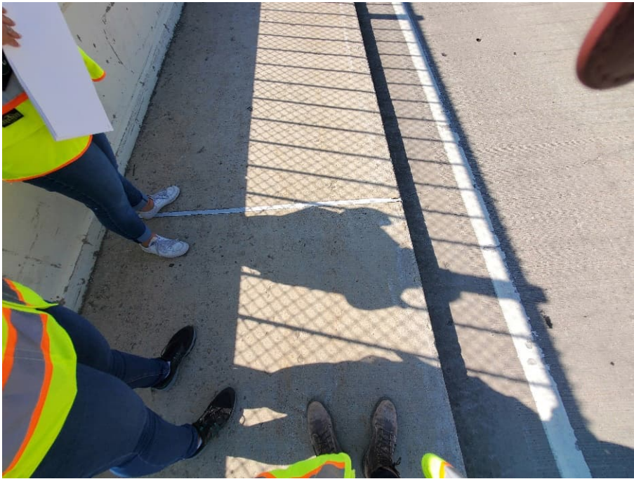
Deck cracking
