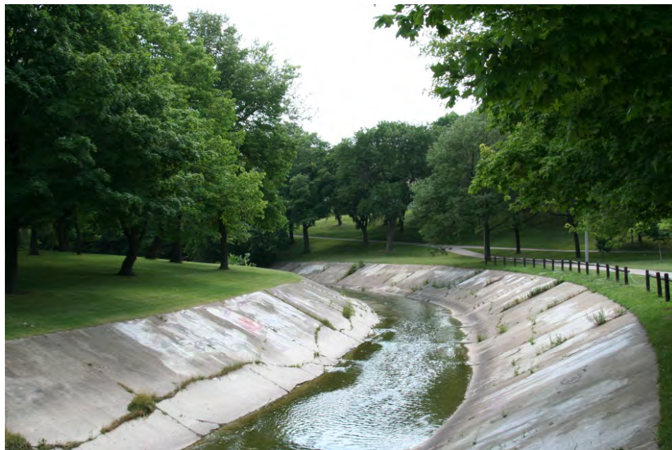
Kinnickinnic River with concrete liner.
