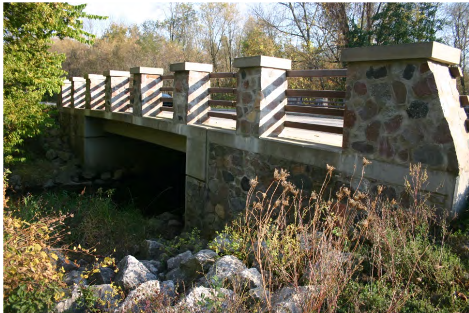
Bridge (c.2000) over Whitnall Creek.
