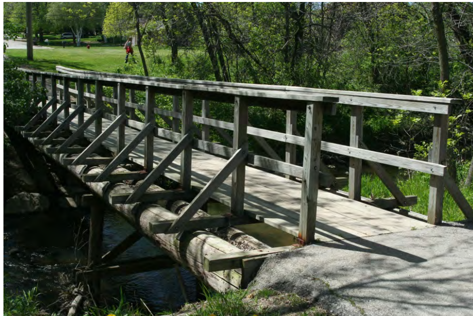
Pedestrian bridge, c.1945, over Oak Creek.
