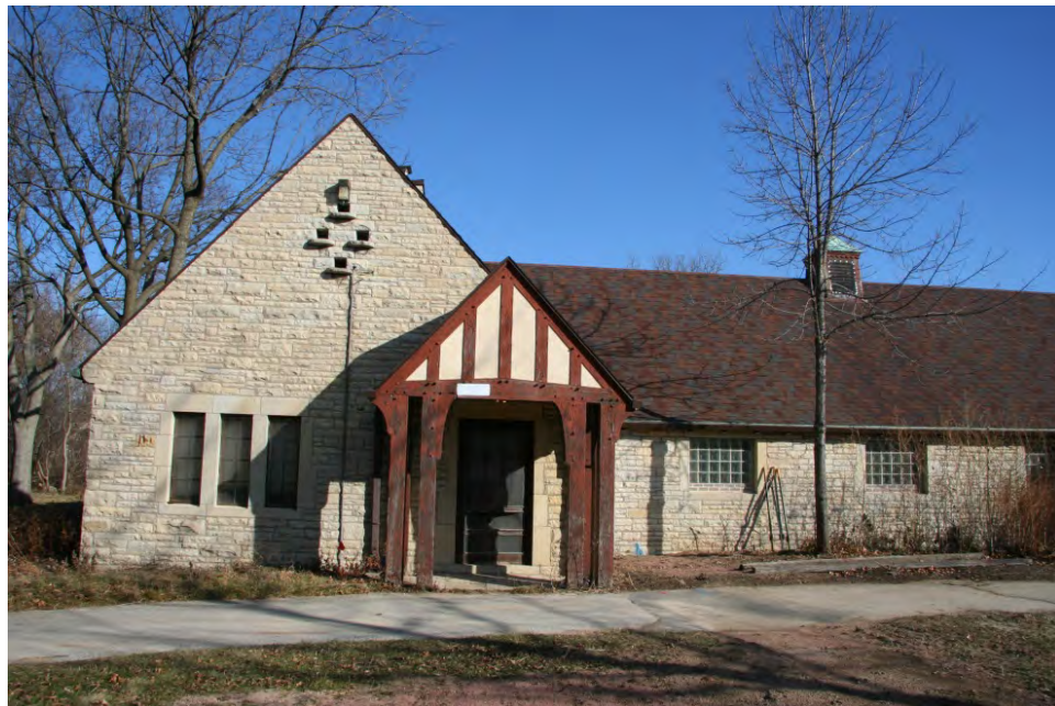
Comfort station in Estabrook Park, constructed c.1937.
