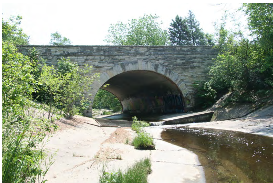
Gault Bridge, constructed in 1933, carries the parkway drive over Honey Creek.
