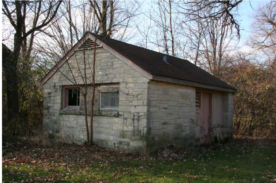
Comfort station located in Lincoln Park Golf Course, constructed c.1952.
