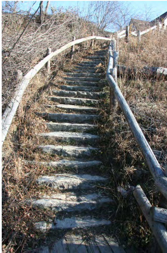
Stone staircase located in Estabrook Park.
