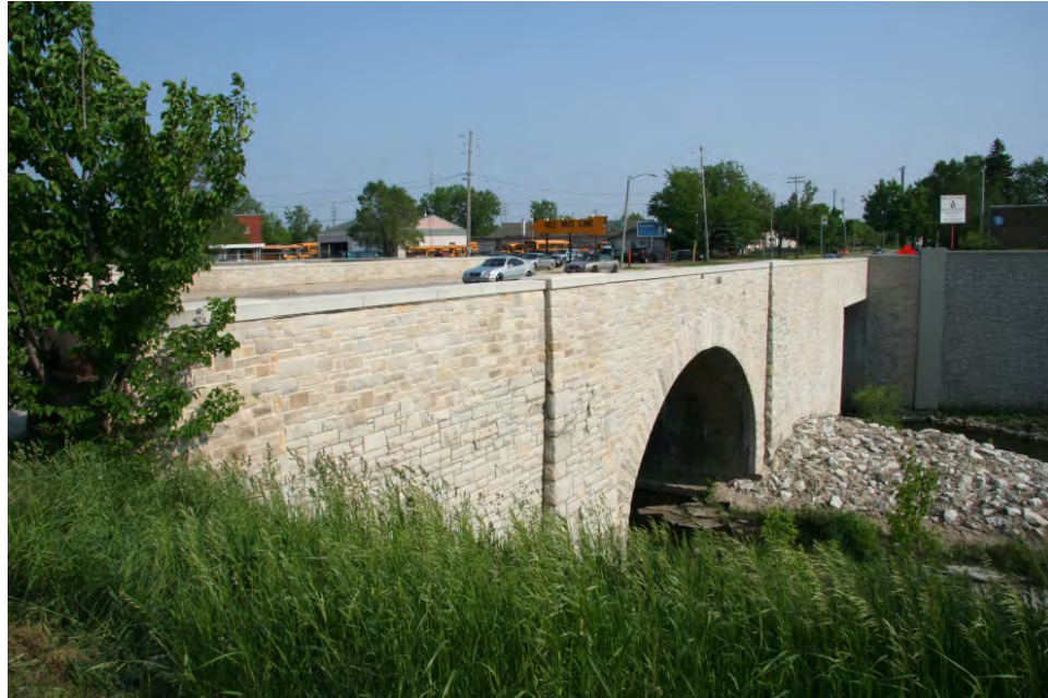
Bridge P-40-0850, constructed in 1937 (left), and a box culvert constructed c.2005 (right), carrying North 35 th Street over Lincoln Creek.
