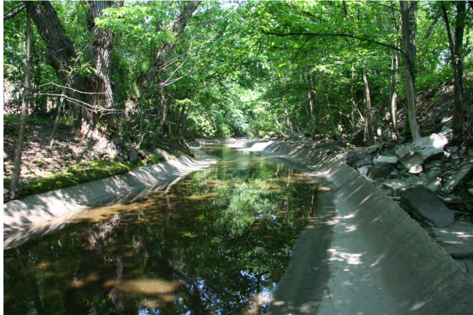
Concrete lined portion of Honey Creek north of West Wisconsin Avenue.
