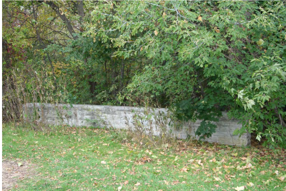
Stone culvert parapet, constructed c.1935.
