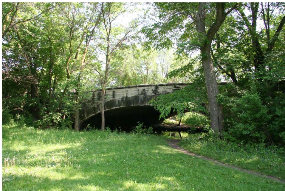
East North Avenue Bridge (B-40-0999), constructed in 1934.
