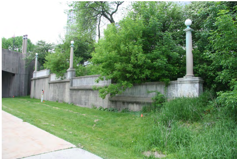
Decorative retaining wall and light standards along Lincoln Memorial Drive, east of Juneau Park.
