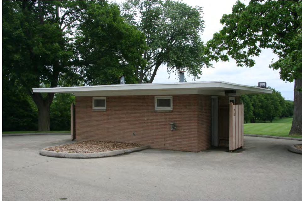
Greenfield Park Golf Course comfort station, constructed in 1957.
