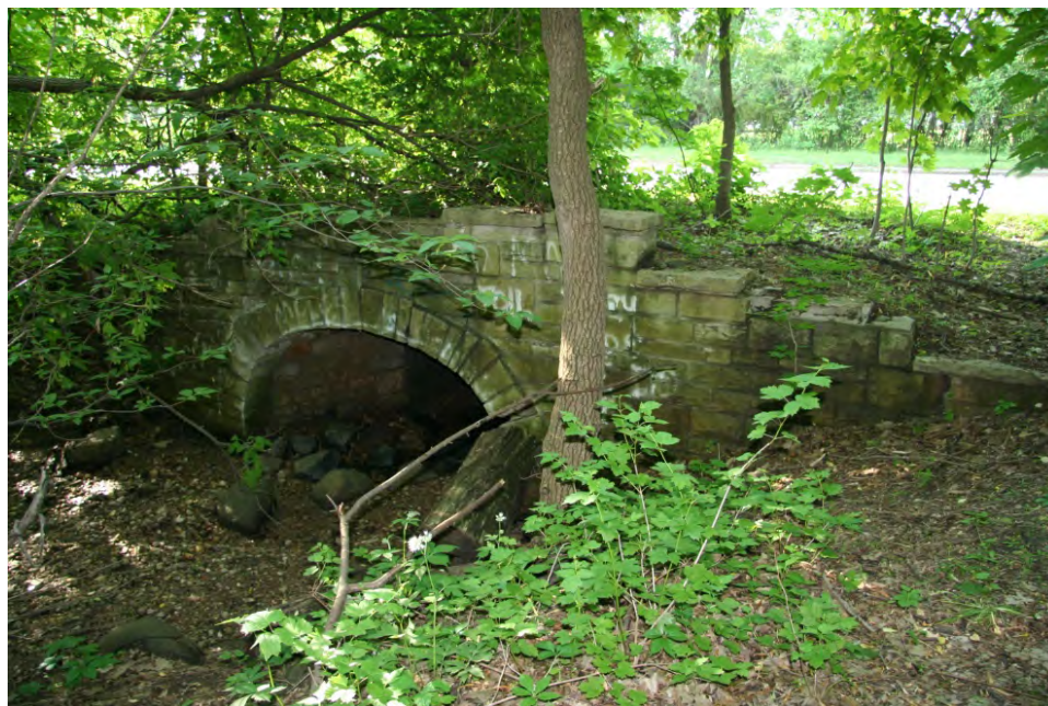
Stone culvert in Jacobus Park, constructed c.1935.
