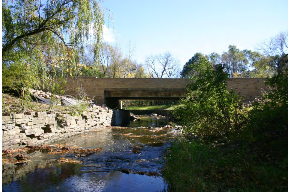
Retaining wall along Honey Creek.
