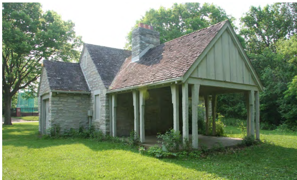
Comfort station, constructed in 1940.
