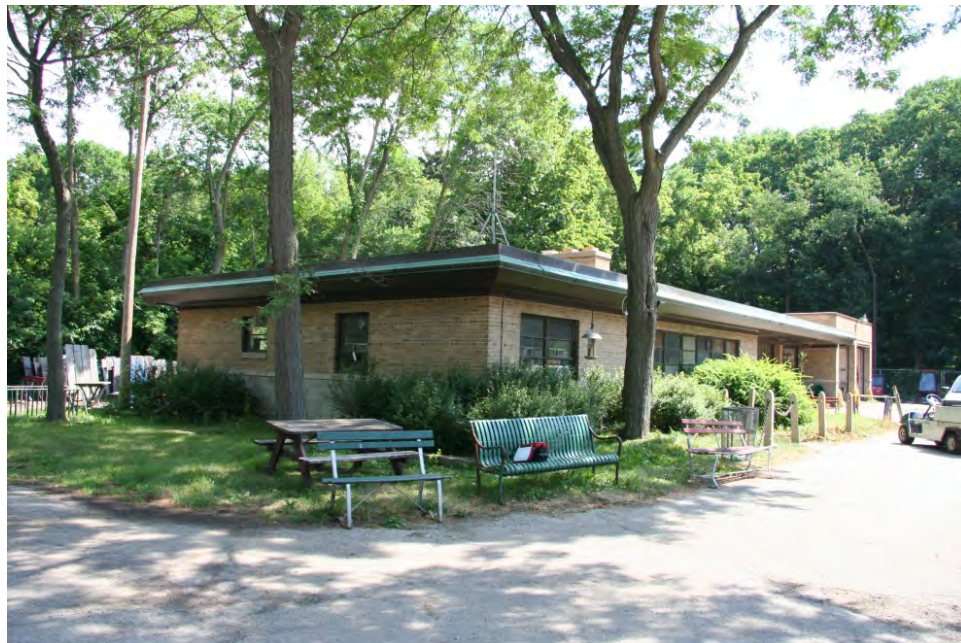
Service and maintenance building in Grant Park, constructed in 1955.
