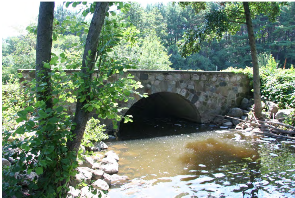
1933 bridge over Whitnall Creek.
