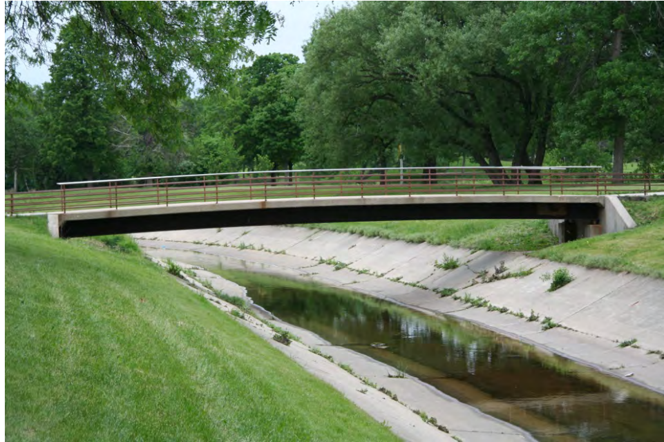
Pedestrian bridge, c.1955, located over Honey Creek.
