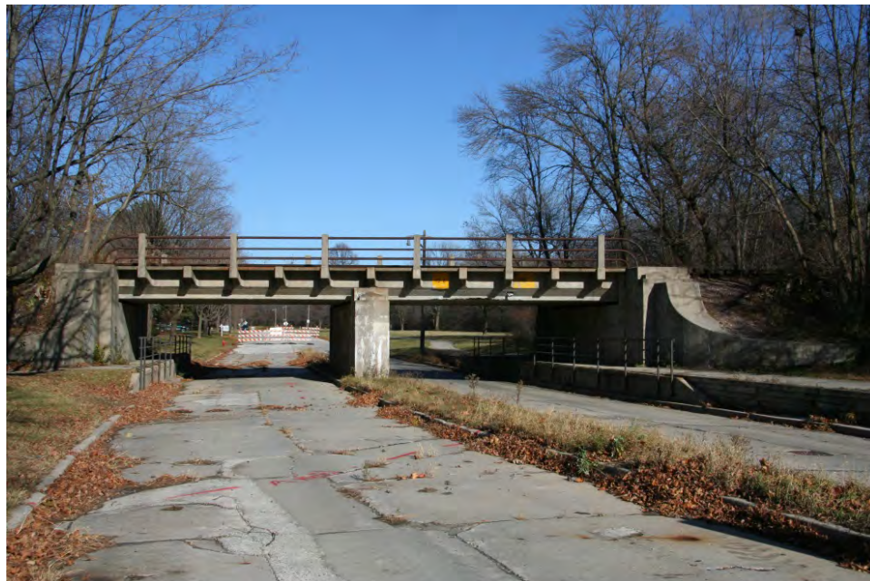
Chicago & North Western Railroad Bridge over the parkway drive, constructed c.1930.
