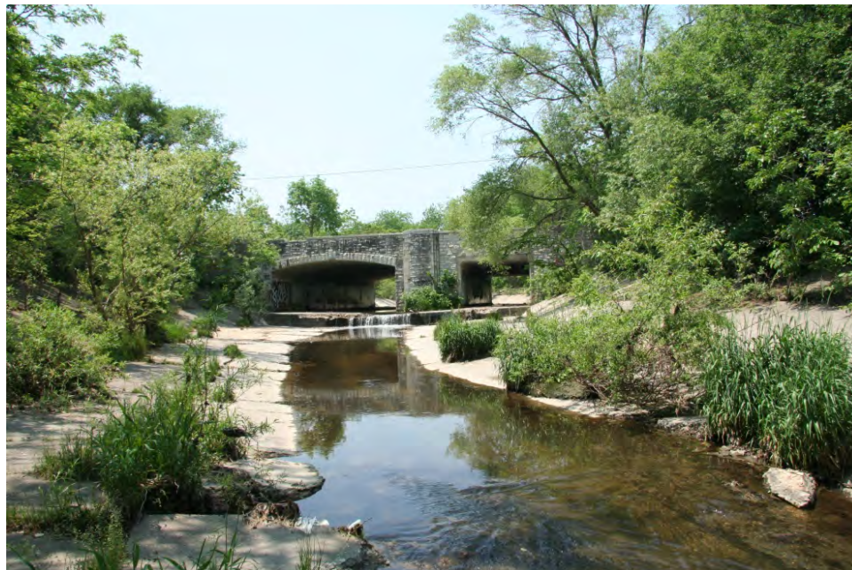
Bridge B-40-0986 and culvert C-40-0016, constructed in 1941 by the WPA.
