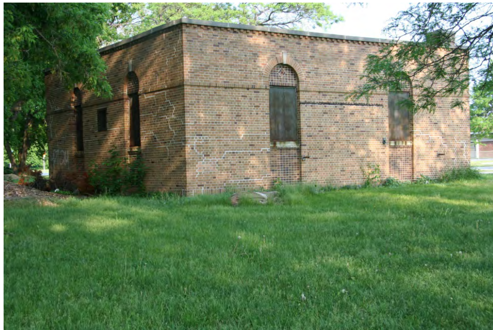
1926 service building in Meaux Park.
