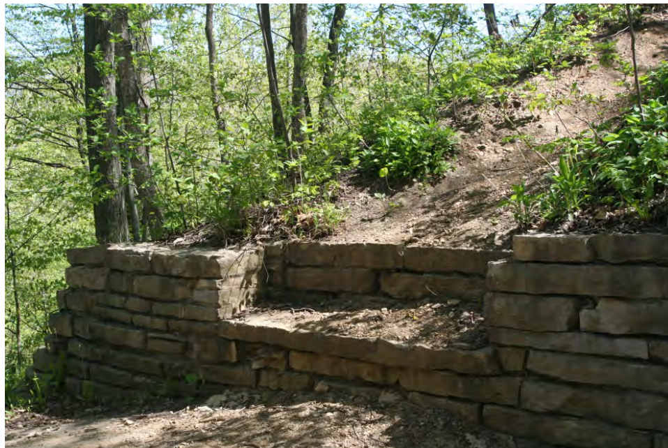
Retaining wall with stone bench.
