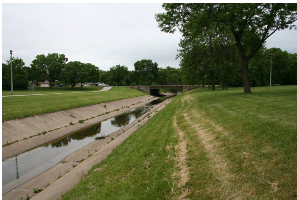
Concrete-lined Honey Creek within the park.
