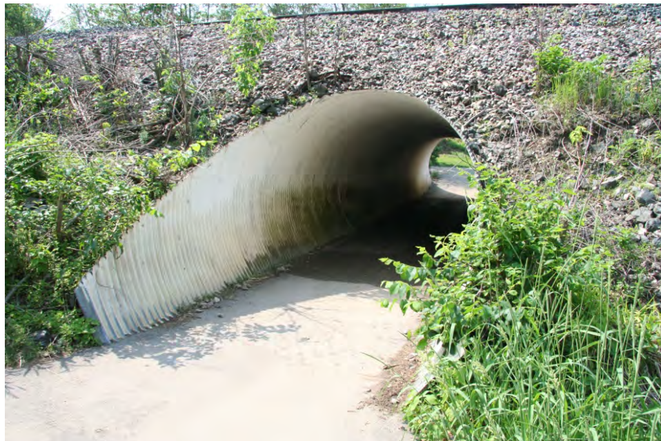
Pedestrian and golf cart tunnel (c.1979) beneath the Canadian Pacific Railroad.
