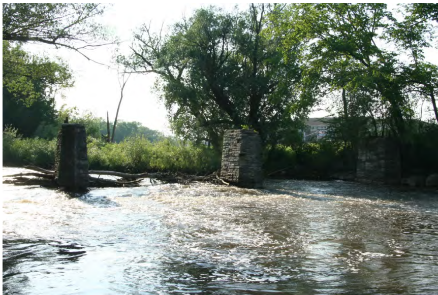
Former bridge piers in the lower segment of the Menomonee River Parkway.
