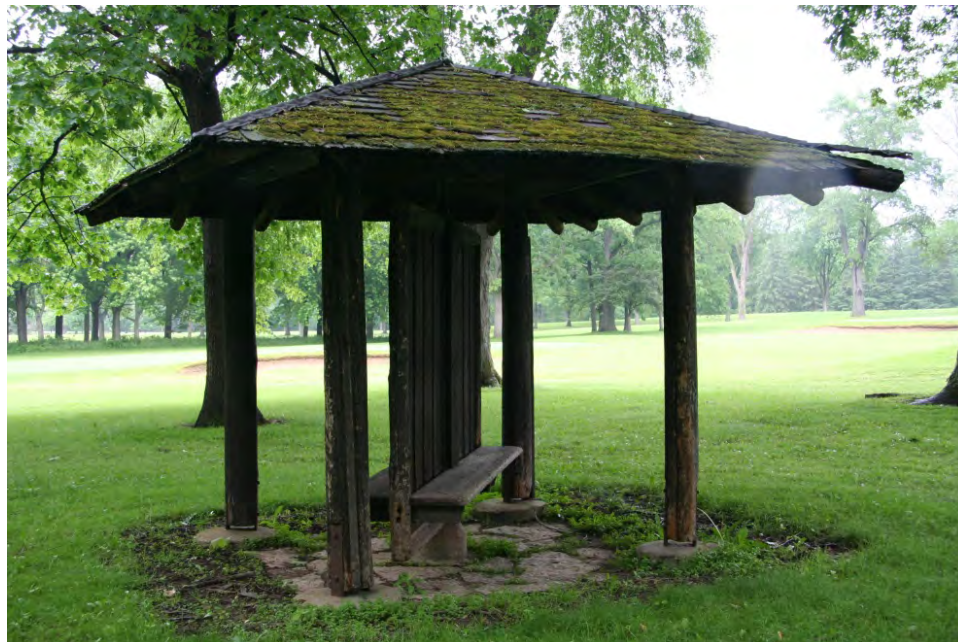
Wood shelter in Whitnall Golf Course.
