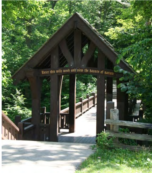
Pedestrian bridge in Grant Park, constructed c.1936.
