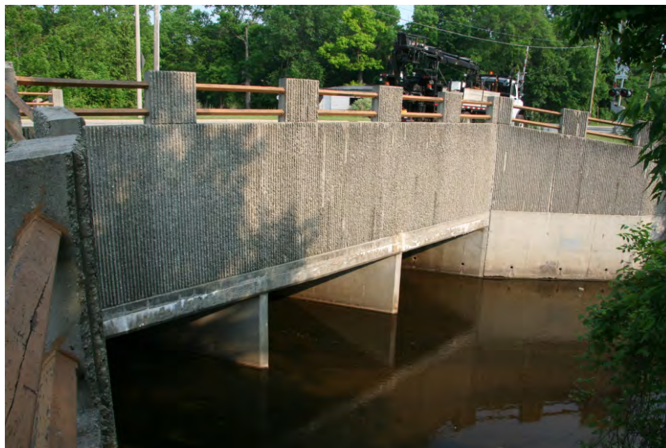
Bridge carrying 115 th Street over Underwood Creek, constructed in 1976.
