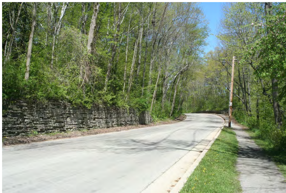
Oak Creek Parkway Drive and an adjacent retaining wall.
