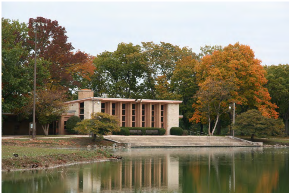
Jackson Park comfort station/community center, also known as the boathouse, constructed c.1960.
