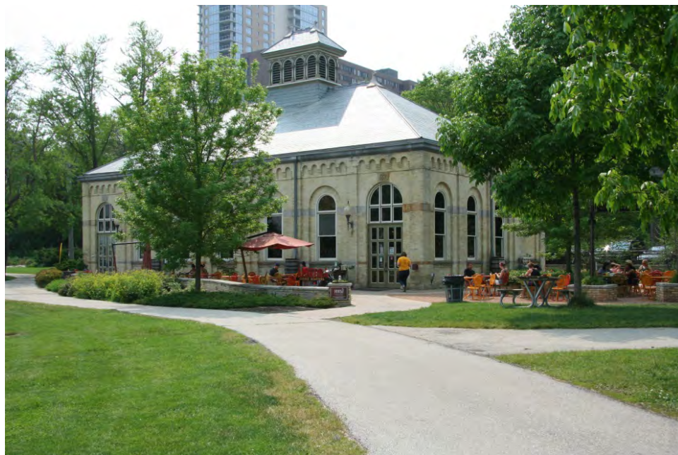
Flushing Tunnel Station, constructed in 1888.
