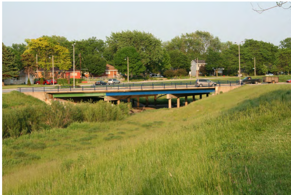
Bridge P-40-0854, 1958, carrying North 60 th Street over Lincoln Creek.
