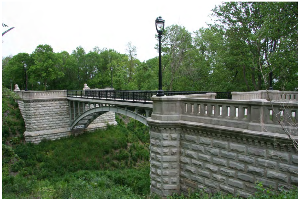
Lion Bridge in Lake Park, constructed in 1896-1897 and recently rehabilitated.
