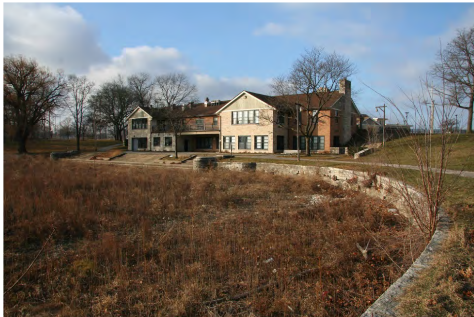
Emil Blatz Pavilion located in Lincoln Park and constructed in 1954.
