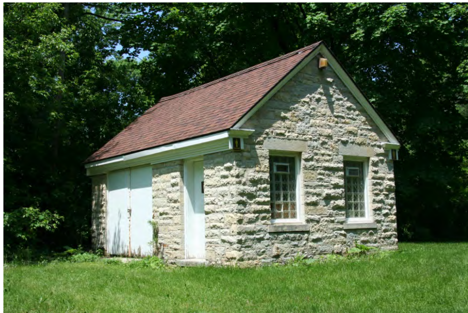
Comfort station in the upper parkway segment, constructed in 1938.
