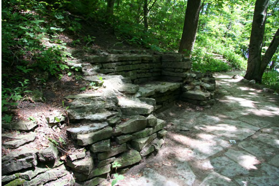
Stone retaining wall with bench in Grant Park.
