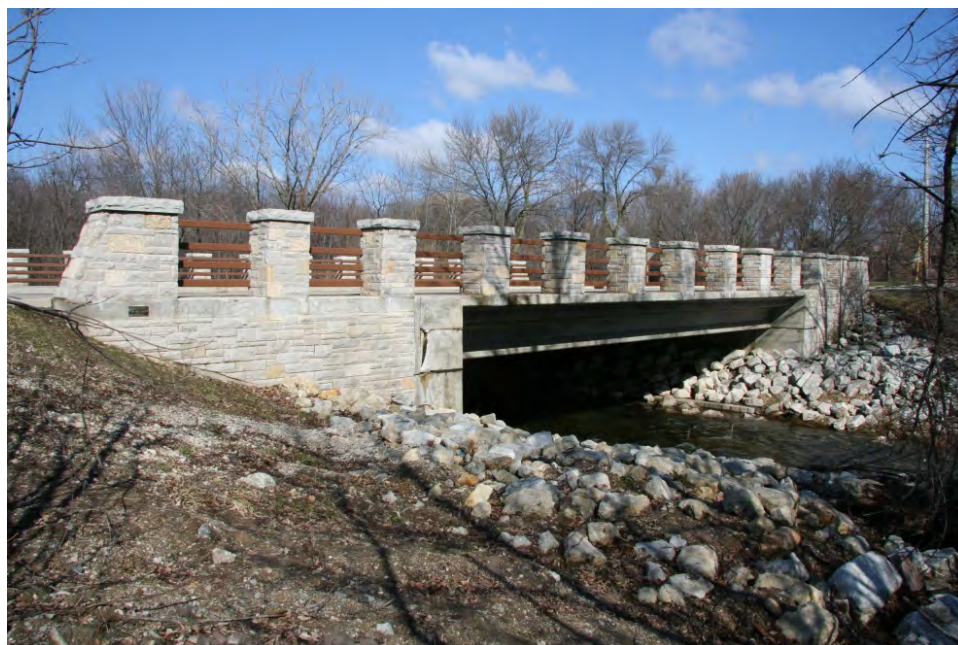
Bridge B-40-0672, constructed in 2002, carries 16 th Street over Oak Creek.
