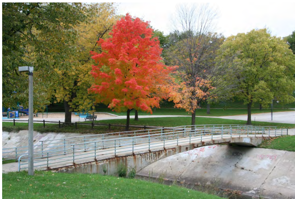
Pulaski Park pedestrian bridge, constructed c.1965.
