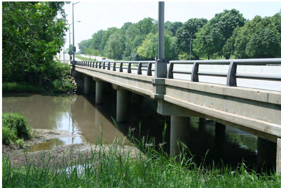
1968 bridge carrying Mayfair Road (STH 100) over the Menomonee River.
