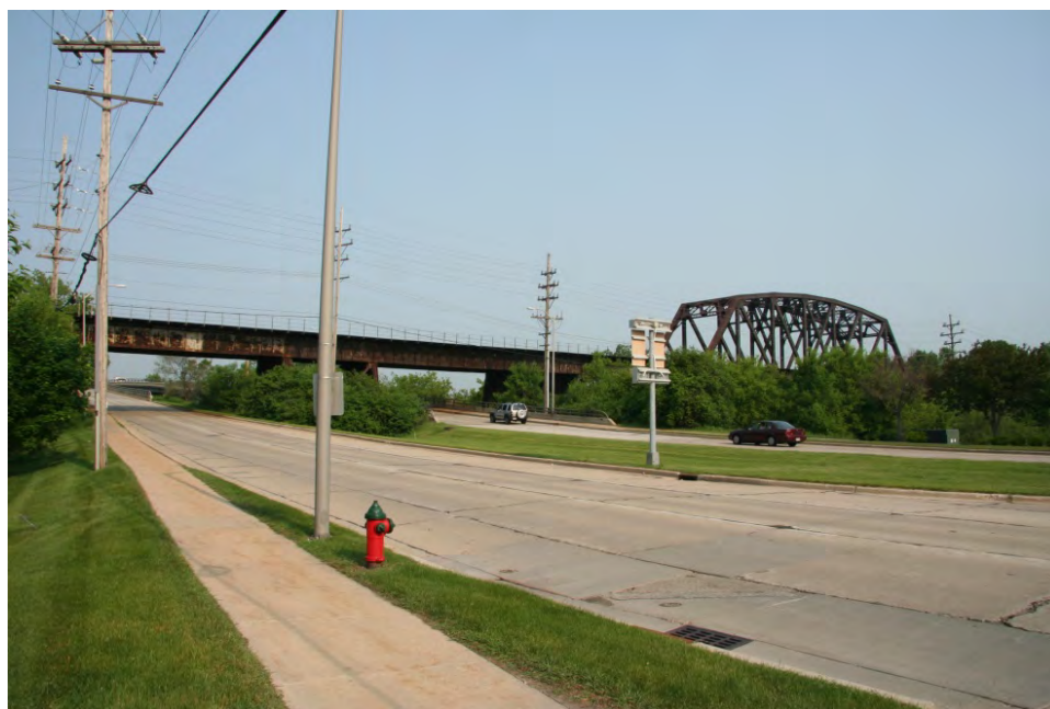
Chicago & North Western Railroad corridor spans the parkway.
