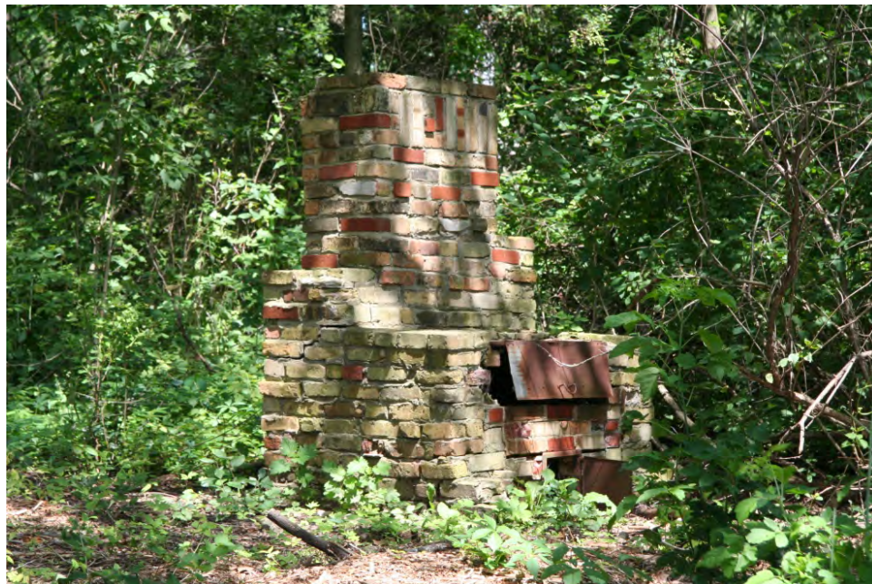
Stone fireplace near the barn in Whitnall Park.
