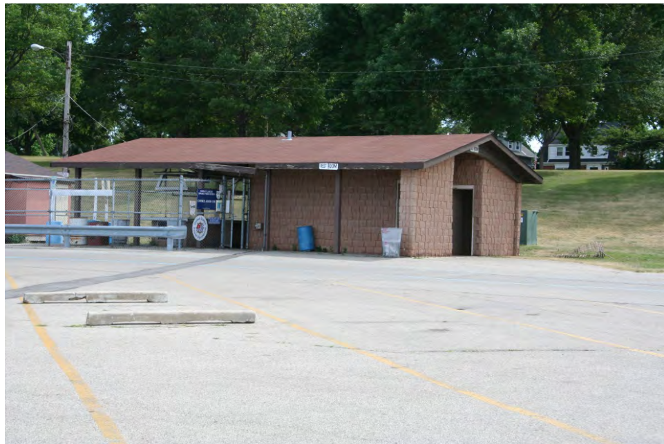
Fish cleaning station with attached comfort station, constructed in 1987 in South Shore Park.
