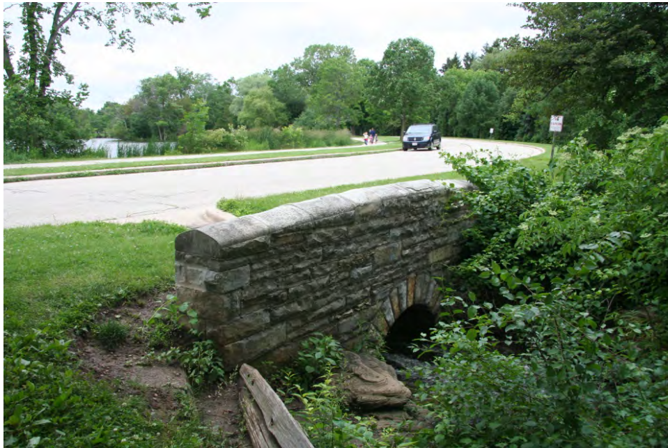
Limestone bridge carrying Park Drive over the lagoon outflow, constructed c.1930.
