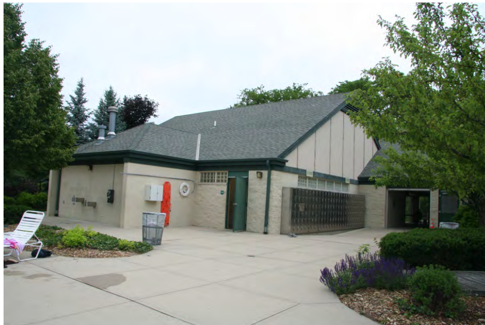
Pool concession stand and changing rooms, constructed in 1997.
