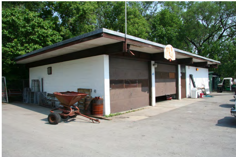
Hansen Golf Course maintenance building (c.1965).
