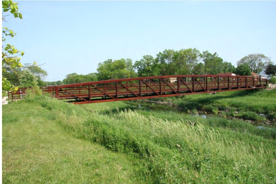
Typical pedestrian bridge, of which there are four located throughout the parkway.
