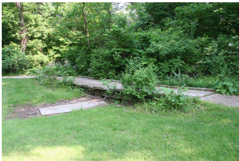
Pedestrian and golf cart bridges in Hansen Golf Course.
