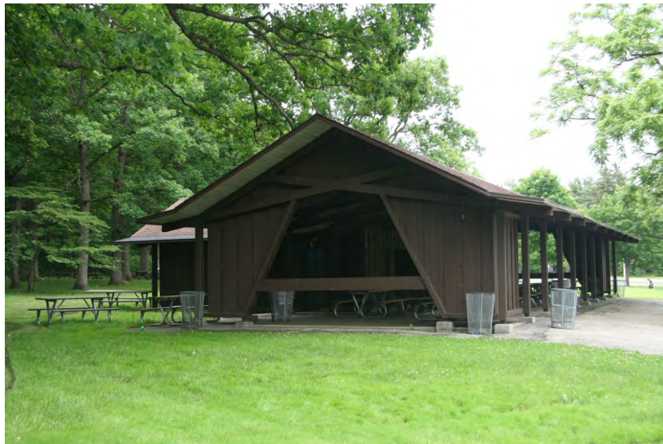
Picnic Shelter with attached comfort station, constructed in 1968.
