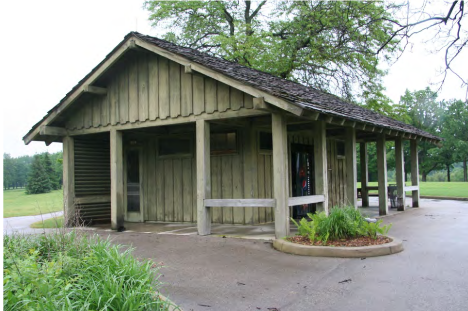
Whitnall Golf Course comfort station, constructed c.1940.
