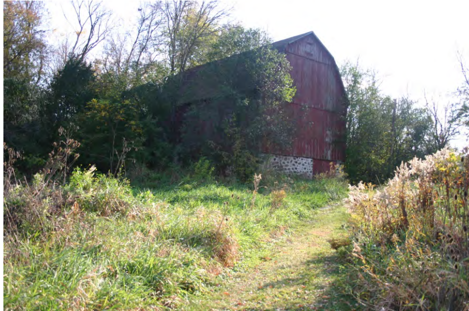
Gambrel roof barn (c.1900) in Whitnall Golf Course.
