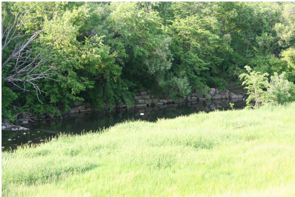
Retaining wall along the east bank of Lincoln Creek.
