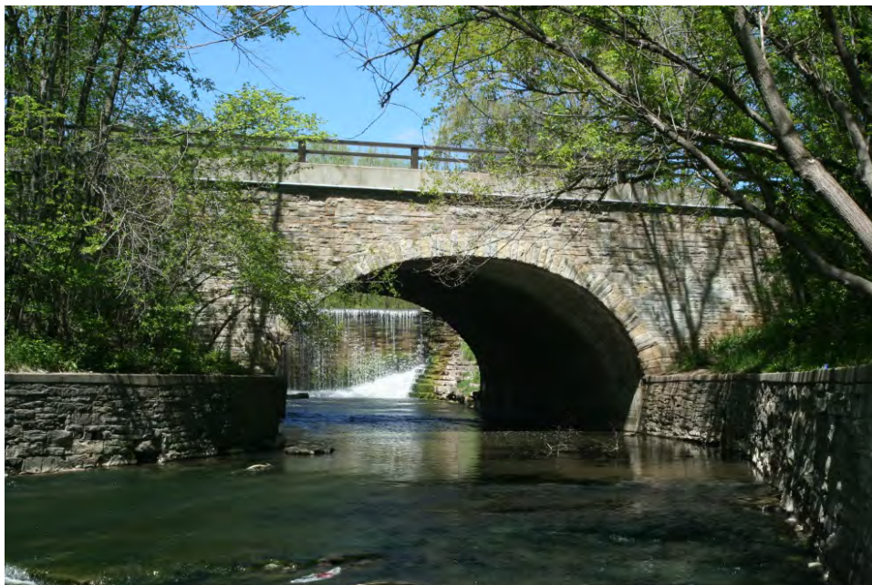
Bridge P-40-0740, constructed c.1931, carries 6 th Street over Oak Creek. The dam is visible in the background.
