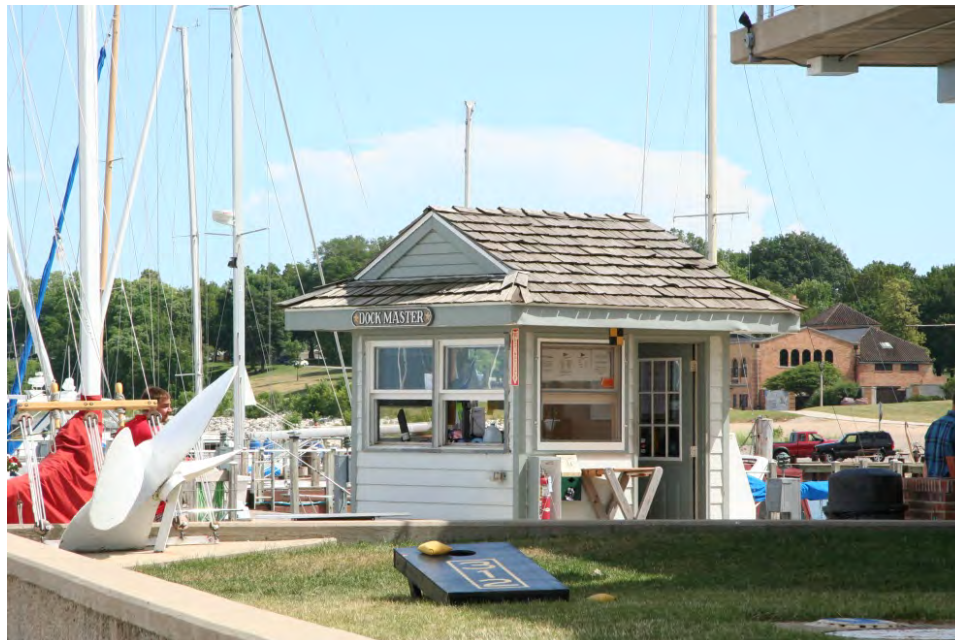
South Shore Park dock operator's house, constructed c.2000.
