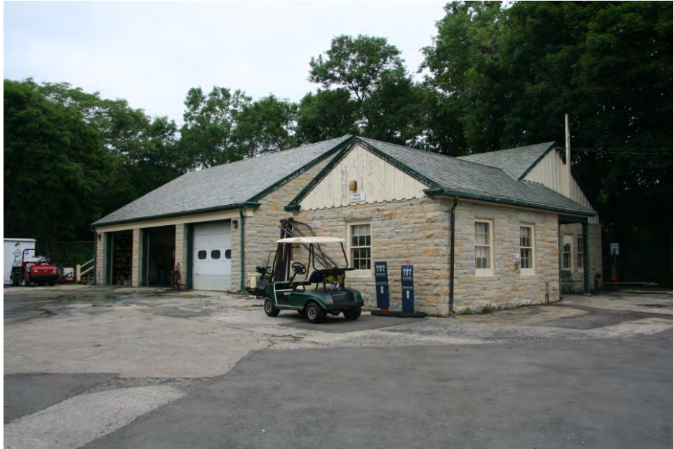
Service building with attached comfort station (not visible), constructed c.1935.
