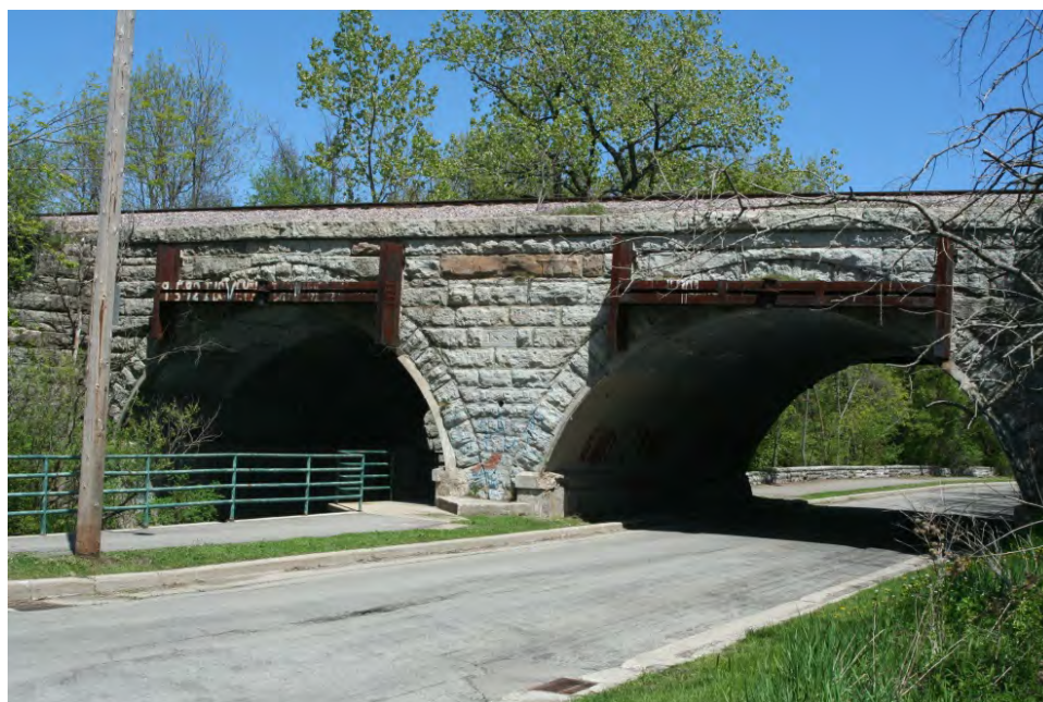
Railroad bridge over the parkway drive and creek, constructed in 1890 with alterations c.1935.
