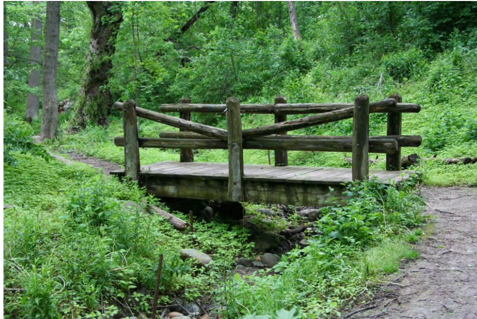
Typical wood pedestrian bridge found in Lake Park.
