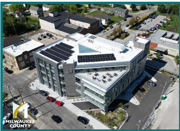
Marcia P. Coggs building with rooftop solar panels and terrace
