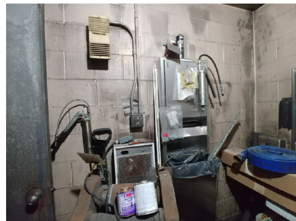
INTERIOR VIEW OF EXISTING RESTROOM
