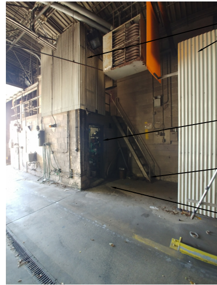
VIEW OF EXISTING RESTROOM WITH MEZZANINE ABOVE
