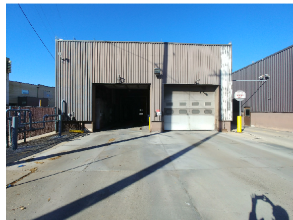
EXTERIOR VIEW OF EXISTING TANK HOUSE (FROM SOUTH)
