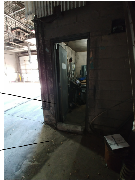
CLOSER VIEW OF DOOR TO EXISTING RESTROOM
