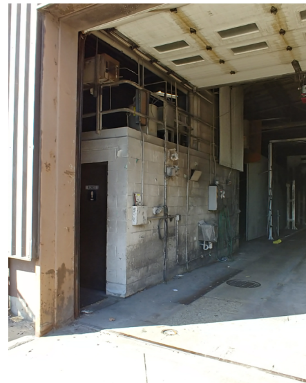
VIEW OF EXISTING RESTROOMS WITH MEZZANINE ABOVE
