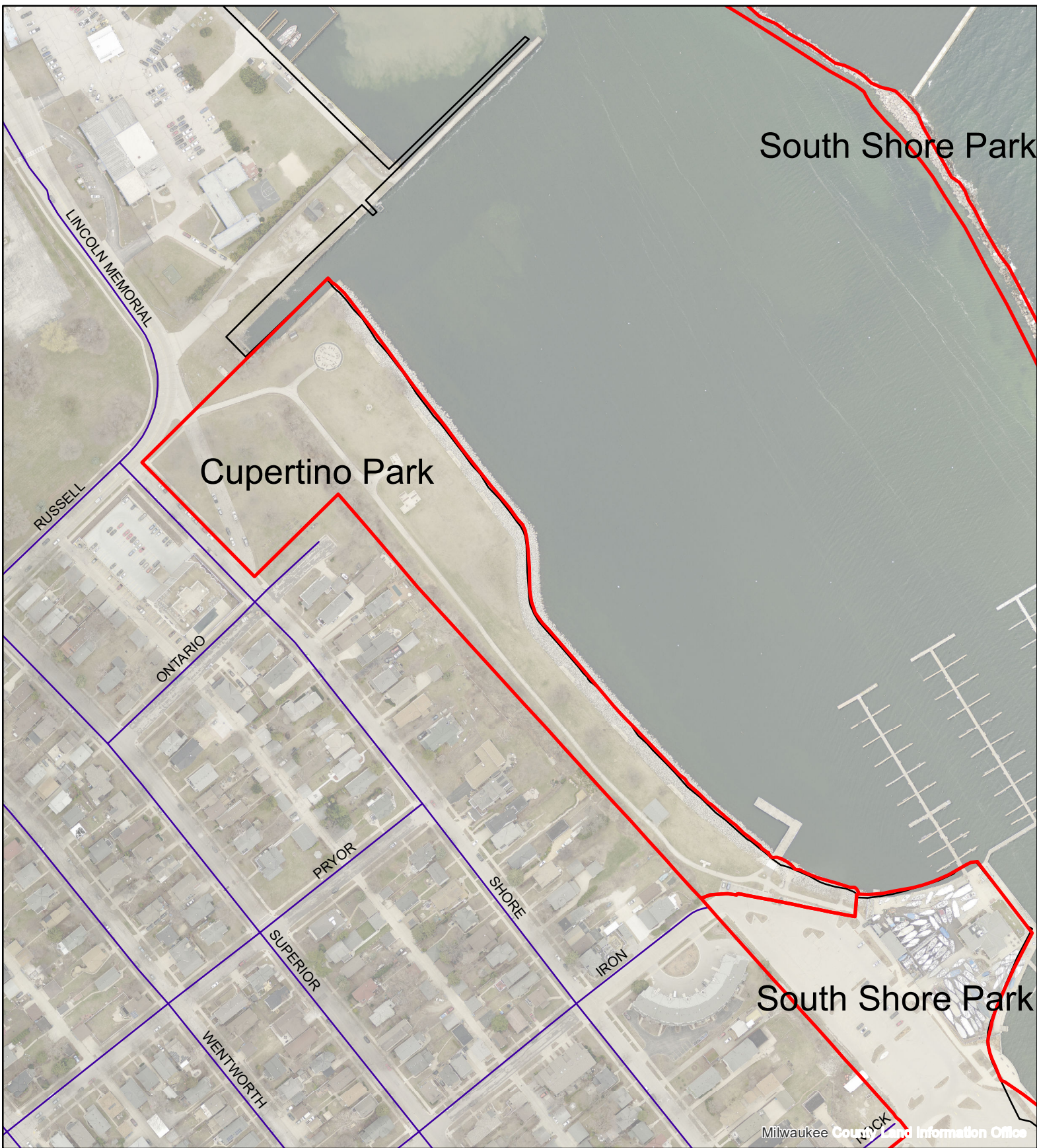
Figure 7 Lake Michigan Bluff Repairs Cupertino Park
