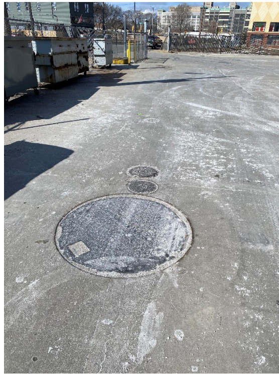
Figure 6: Service Building (North Side) New Oil UST
