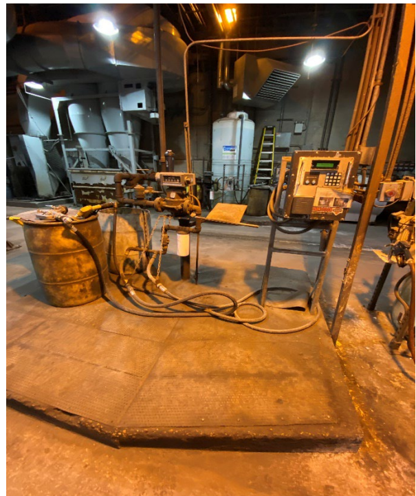
Figure 4: Service Building (North Side) Pumping Station
