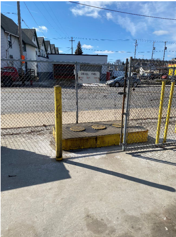
Figure 7: Service Building (North Side) Fill Area
