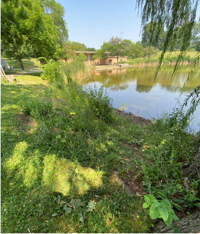
Figure 1: Picture of constructed wetland on northwest side of lagoon.
