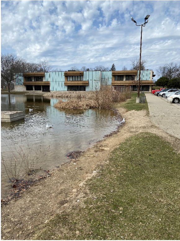
Figure 1: Eroded shoreline on east side of lagoon by parking lot.
