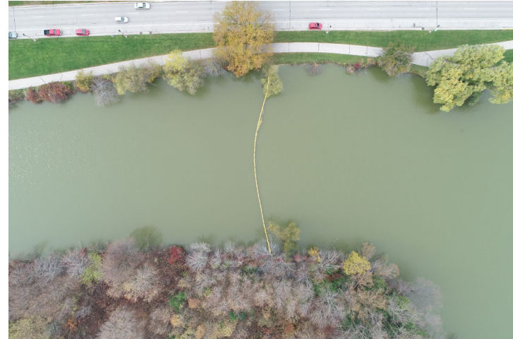
W – View of Turbidity Curtain
