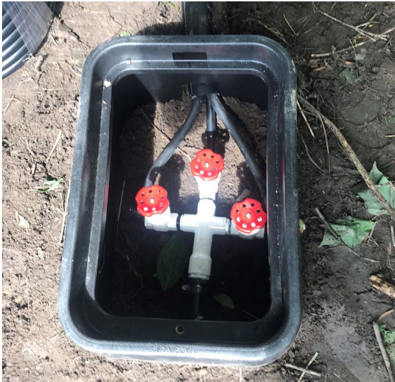
Directionally Bored Conduit and Air Diffuser Manifold
