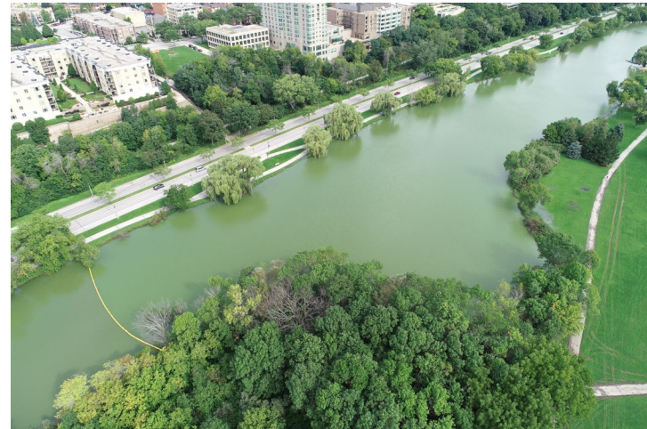
NW – View of Turbidity Curtain/North-End of Lagoon
