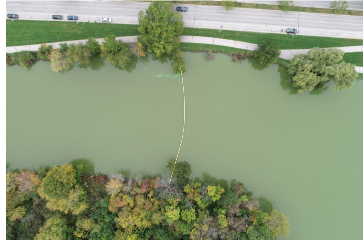
W – View of Turbidity Curtain
