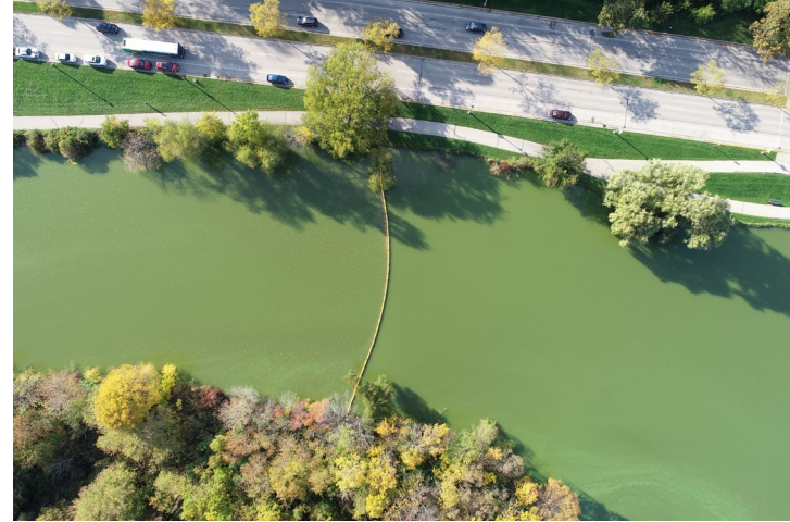
W – View of Turbidity Curtain
