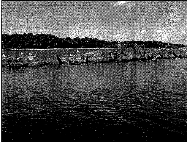
③ OFFSHORE BREAKWATER LOOKING LANDWARD
