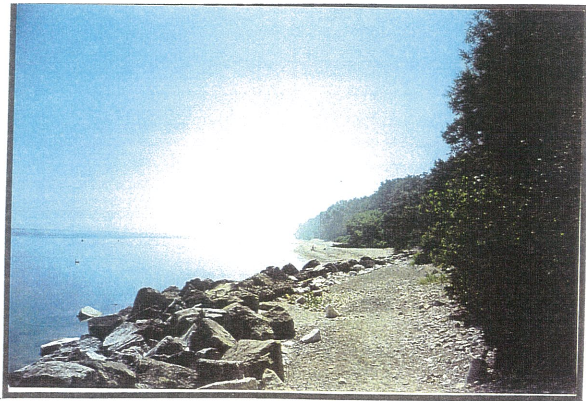
PHOTO #4: SHORELINE FACING SOUTH – NOTICE STONE PROTECTION
