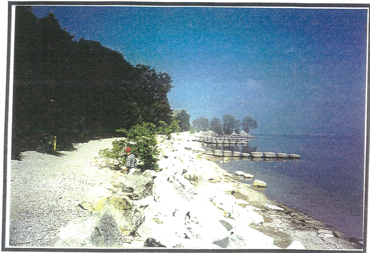
PHOTO #1: SHORELINE SOUTH OF SOUTH SHORE PARK, FACING NORTH. NOTE STONE PROTECTION AND GROINS..
