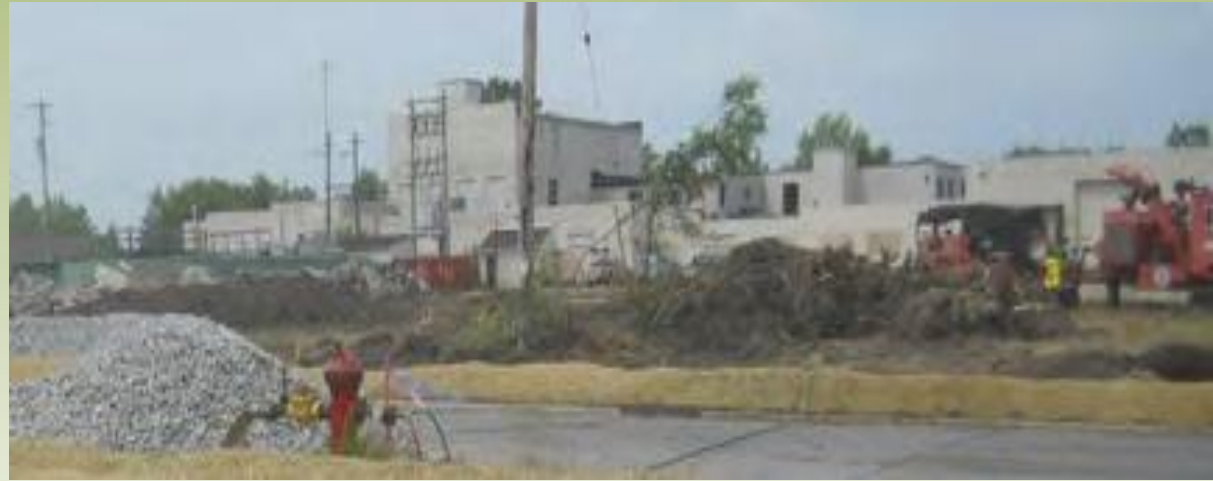
Former Midwest Tanning at 1200 Davis Avenue
