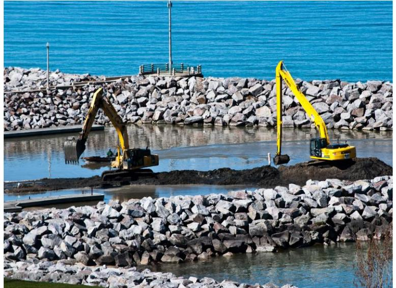
Excavators removing sediment from the boat launch
