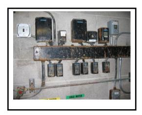
The electrical equipment in the HVAC equipment room appears to be in good condition. It was noticed that the Motor Control Center does not have the required 3ft working clearance in front of the equipment to meet code.
