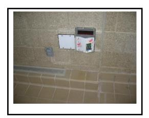
The electrical devices in the pool area are in need of repair. The cover plates are rusted and corroding. The electrical devices in the non-pool area appeared to be in good condition.
