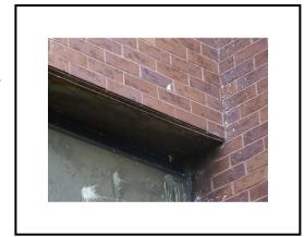
Similar corrosion of the lintel plates is present at the patio doors along the west side of the pool and the conference room windows along the north wall. Similar conditions may exist along the clearstory windows along the east wall of the pool area. These windows were not accessible for inspection.
