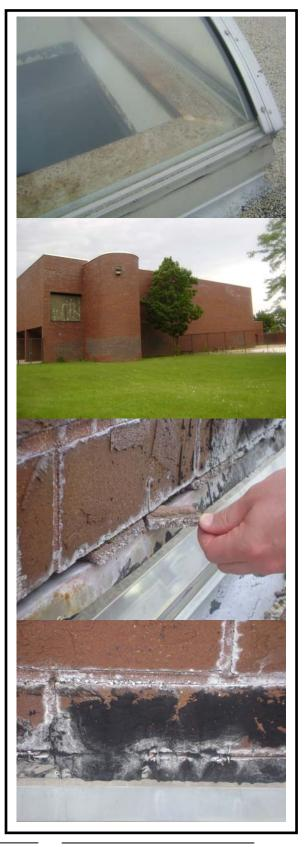
the wall cavity. Thus, as moisture laden air migrates from the interior pool room through the wall to the exterior, the moisture is being deposited within the wall.
