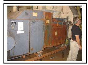
HV-2 is 100% OA system consisting of Trane modular air handler with dual centrifugal fan assembly, heating coil with three way control valve, 30% eff. 2" thick filter section, return fan with relief damper, outside air intake with flat plate heat exchanger and associate face-bypass dampers.
