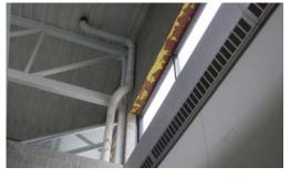
by moisture within the pool air condensing on the cold lintels in the winter and/or water penetrating from the exterior wall. From our visual review and comments for the maintenance staff we believe that the exterior wall is the main culprit and will need to be repaired prior to the lintels being repaired and repainted. Most likely this wall is also causing the damage/leaks in the ceiling in the lobby.
