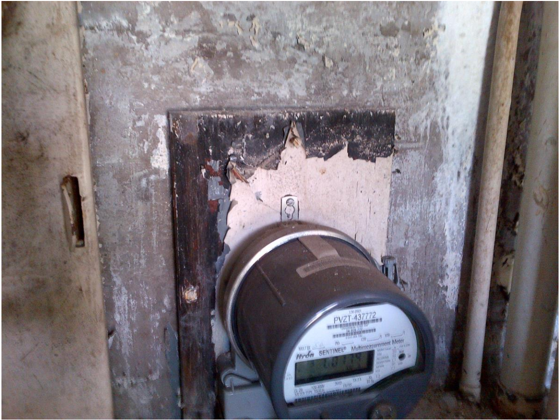
PHOTOGRAPH NO. 7: Subject Property –meter
