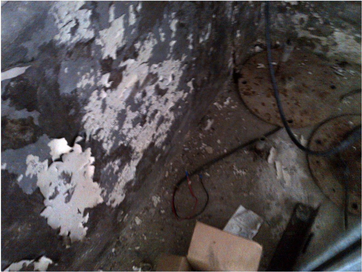
PHOTOGRAPH NO. 5: Subject Property – floor of building
