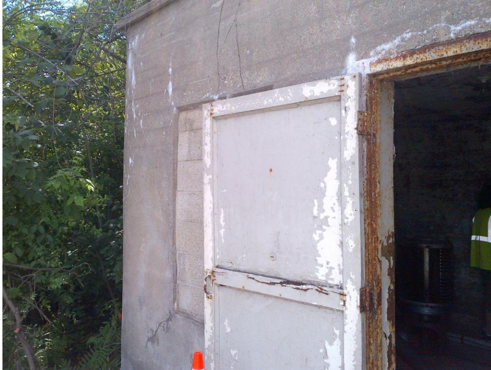
PHOTOGRAPH NO. 1: Subject Property – Exterior Door
