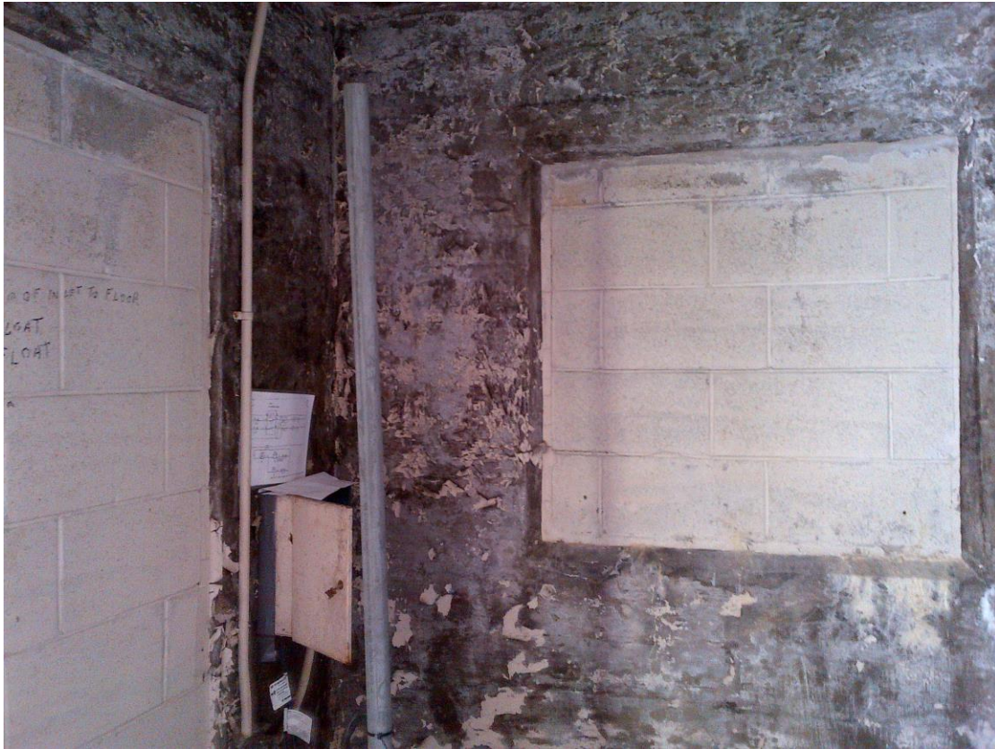
PHOTOGRAPH NO. 3: Subject Property – east wall
